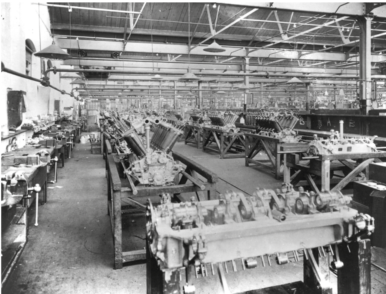
Copyright Rolls-Royce plc: Rolls-Royce Eagle Engine on build at Main Works, First World War.
