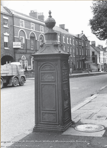
Electrical transformer kiosk, Friar Gate, 1970's - these formed part of Derby's original electrical lighting scheme of 1893 (Picture courtesy of Derby City Council).
